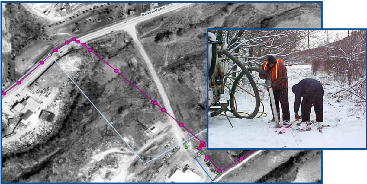
TSH/TBE mapped 12 km of water infrastructure
