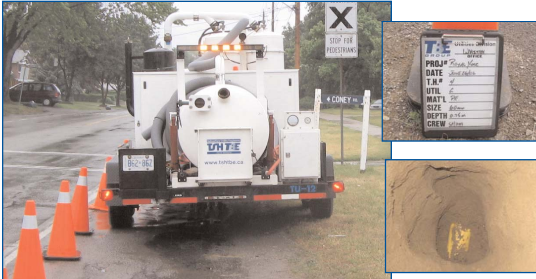
Utility Investigation along Royal York Road
