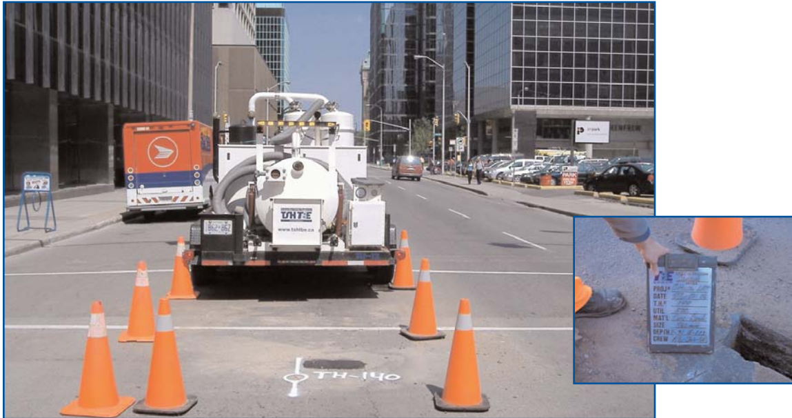
Utility Investigation along Albert Street and Slater Street
