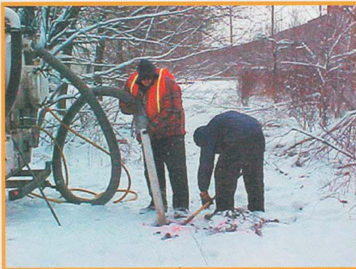
Photo #1: Field crews completing test holes during winter conditions.
