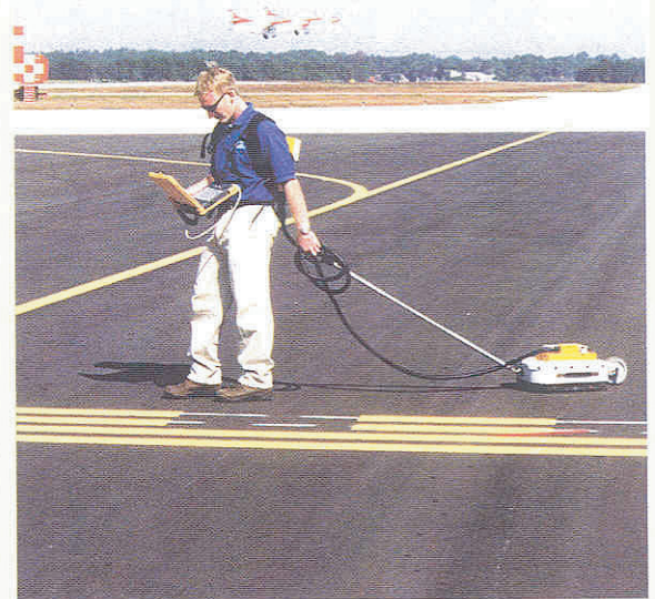
Ground Penetrating Radar (GPR) used to obtain QL - B information at an airport.
