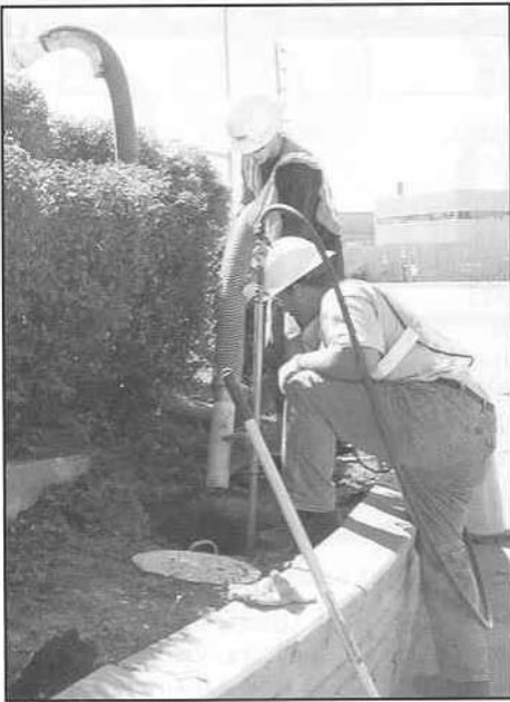
SUE Technicians installing a test hole at the intersection of Airport Road and Derry Road in Mississauga, Ontario.
