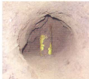
A SUE test hole exposes an underground gas main.
